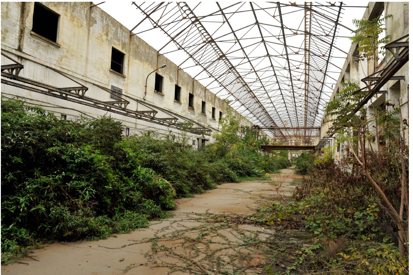
Fig.75:Internal view of Ex Macello Gallery
