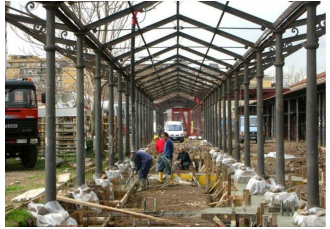
Fig.84: Mattation pavilion. Source: ArchiDiAP - Foundation reinforcement - Source: ArchiDiAP
