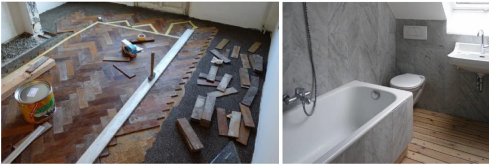
Figure 18: renovation phase of the Warland project
