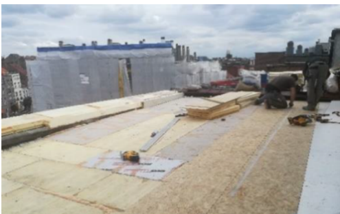
Figure 20: Petite-Suisse renovation process made with over-ordered materials
