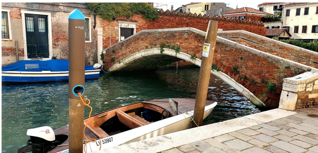
Fig. 2.27 - e-dock column installed.
