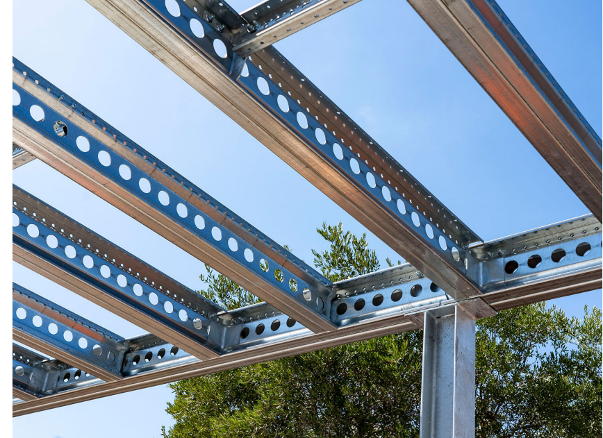
Fig. 4.14 Close up picture of Mechano Steel Frame structures
