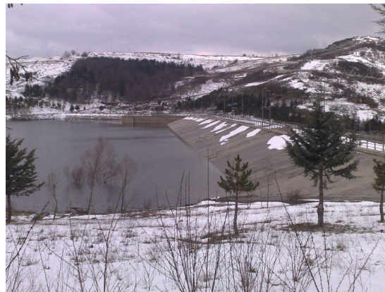
(c) Saetta dam (Basilicata Region).
