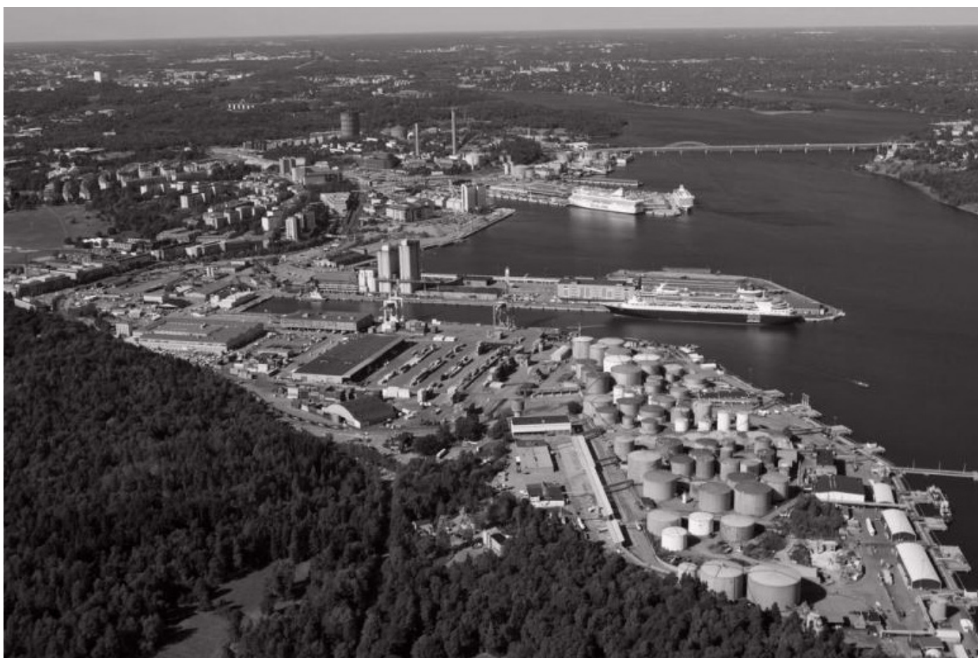
View from the south before the oil tanks were taken down and the container handling was relocated Lennart Johansson
