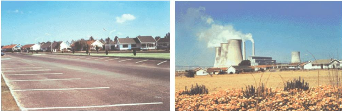
Figure 7-3 Residential houses built for the employees (left), View of the residential property with the power station in the background (right) [62]
