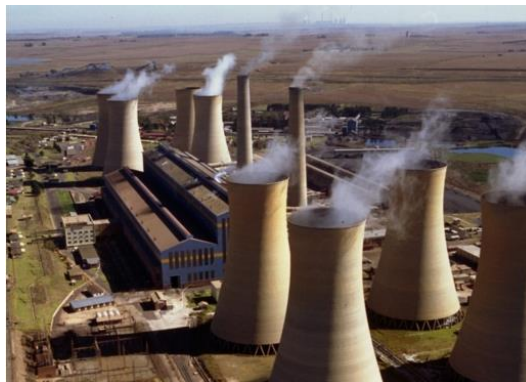
Figure 7-2 Komati power station
