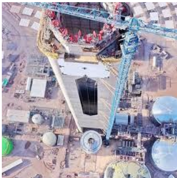
Figure 1-3 Atacama solar tower construction
