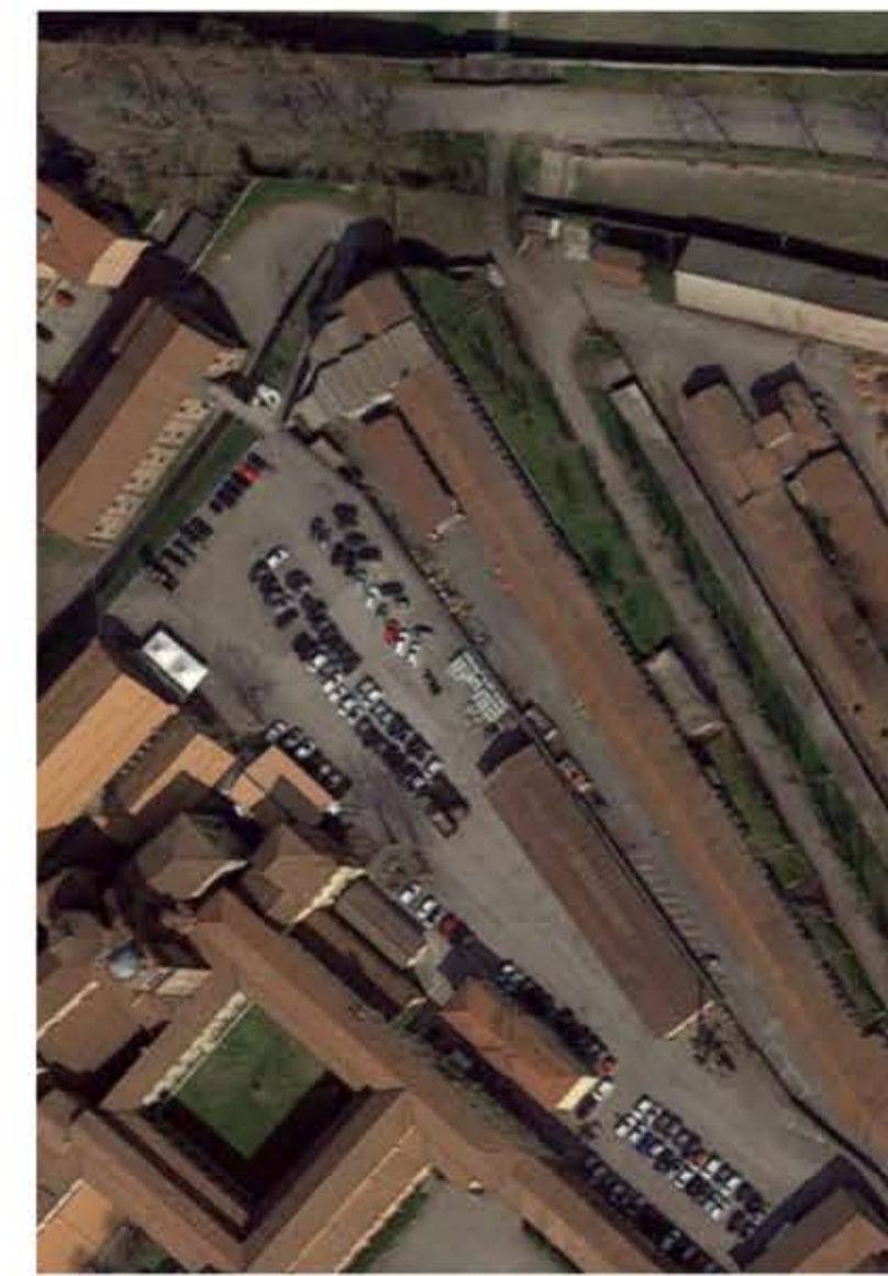
Existing parking space for military personnel inside the caserma Filippo Nicolai with access from Piazza Casali.
