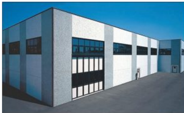
Figure 1.1: Pre-cast structure with cladding panels
