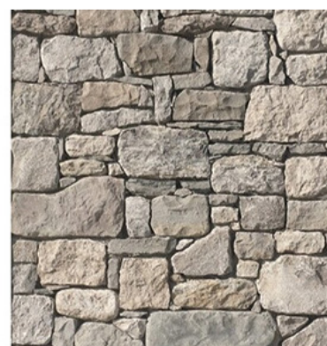
Retaining wall (RW)
