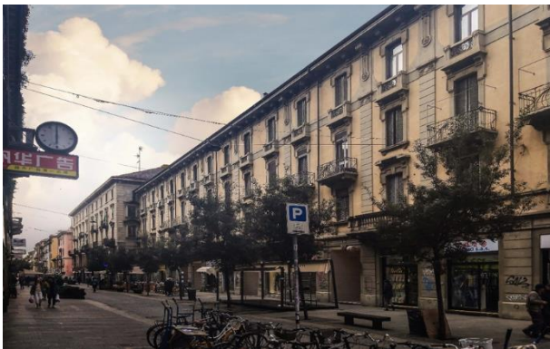
Picture n. 38: The existing facades on Via Sarpi, Niccolini and Bramante will be maintained – https://blog.urbanfile.org/ , 2022
