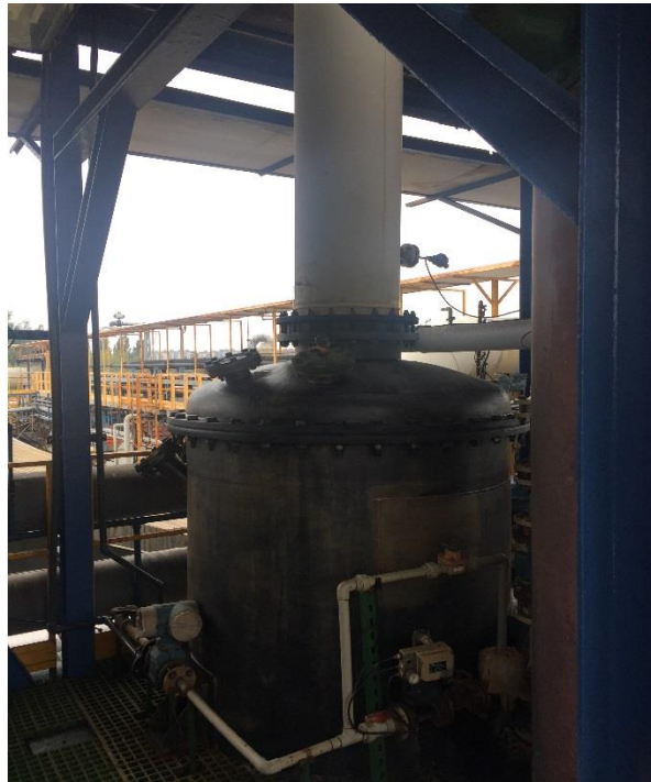
Figure 12.6. Flash column and valve with repaired conditions
