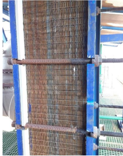
Figure 12.5 Plate and Frame heat exchanger
