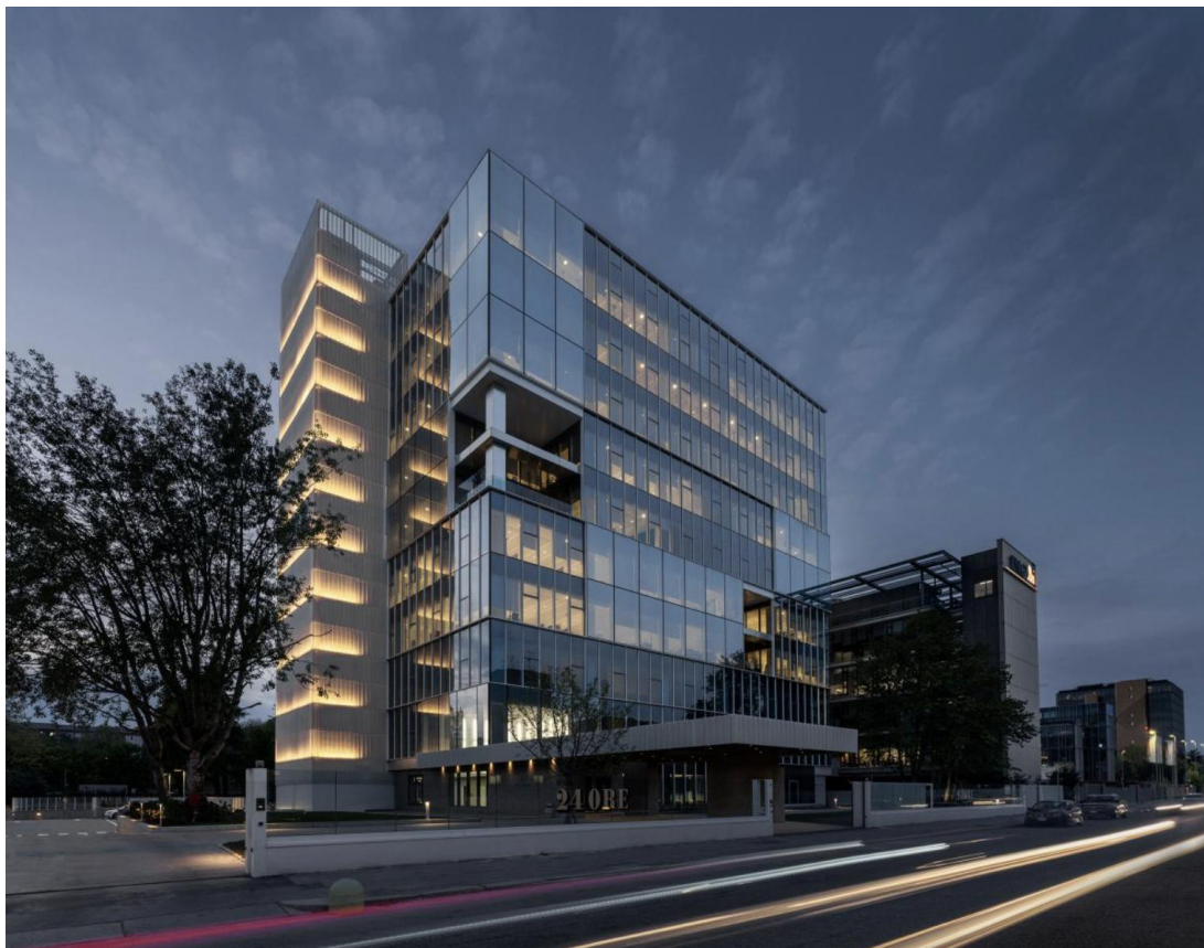
Figure 4-3 – Exterior view and primary façade of the Il Sole 24 office building.
