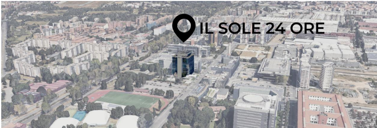
Figure 4-2– Il Sole 24 case study building within the urban context of Milan.
