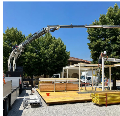
Figure 6: outdoor installation process
