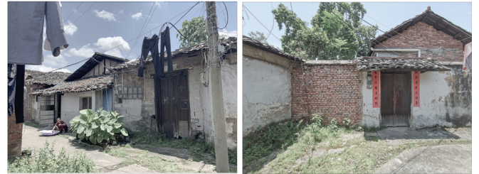
2 | MV: The building was built in modern times, belonging to the common folk houses MQ: The building can be used, the structure is stable, the main components are missing and dilapidated
