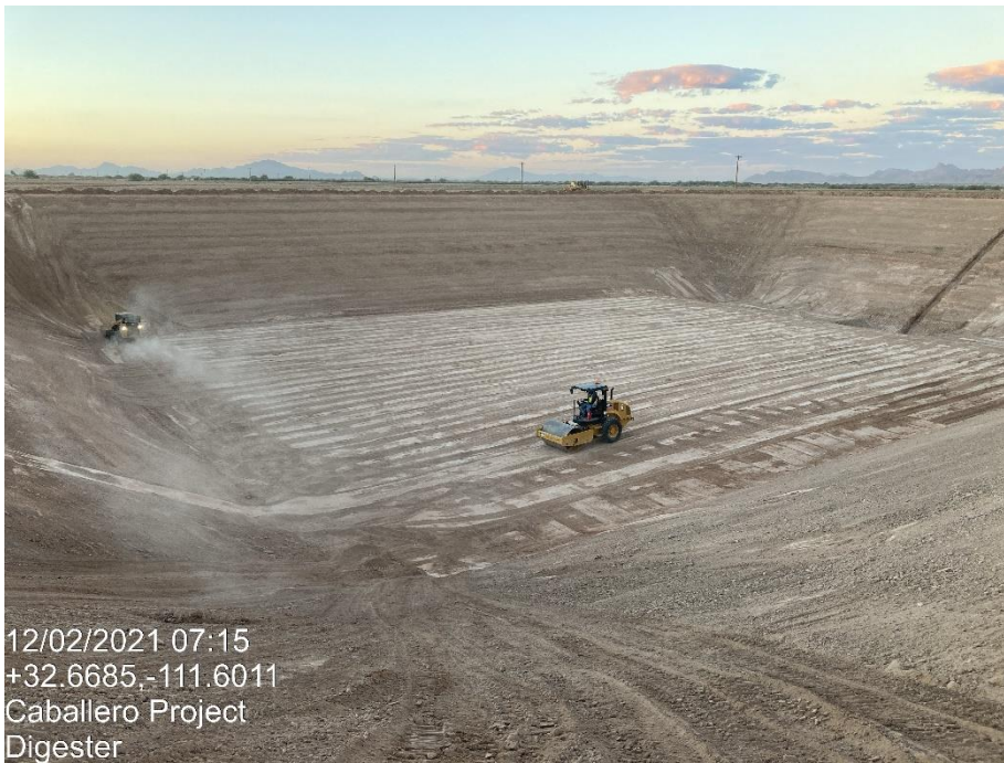
Figure 4.1.3 Lagoon excavation nearing completion
