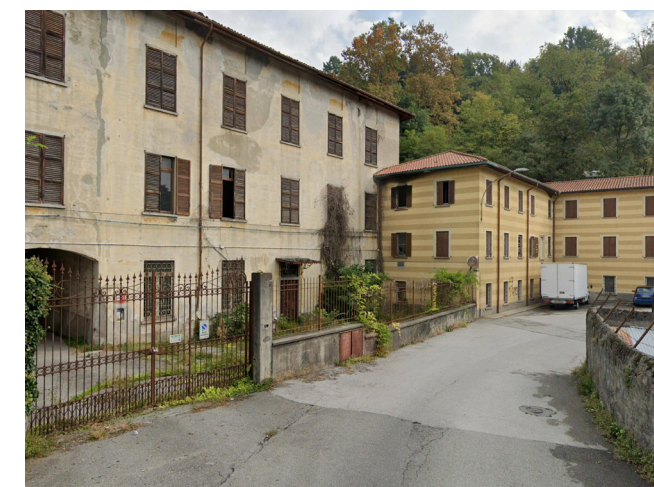
Figure 15 paper mill front view
