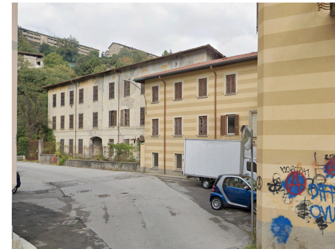
Figure 14 paper mill front view
