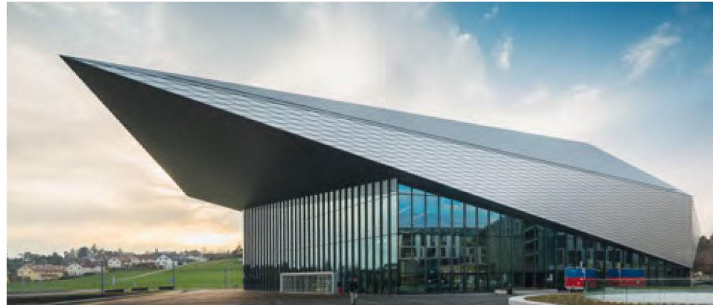
Figure 24 Convention Center, Lausanne, Switzerland
