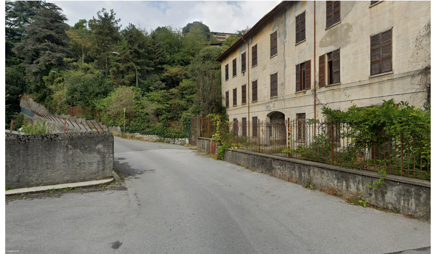
Figure 16 Garabuso road in front of paper mill front view
