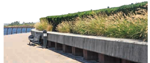
Figure 27 : Flood wall constructed along waterfront walkway Source: southamboynj.gov
