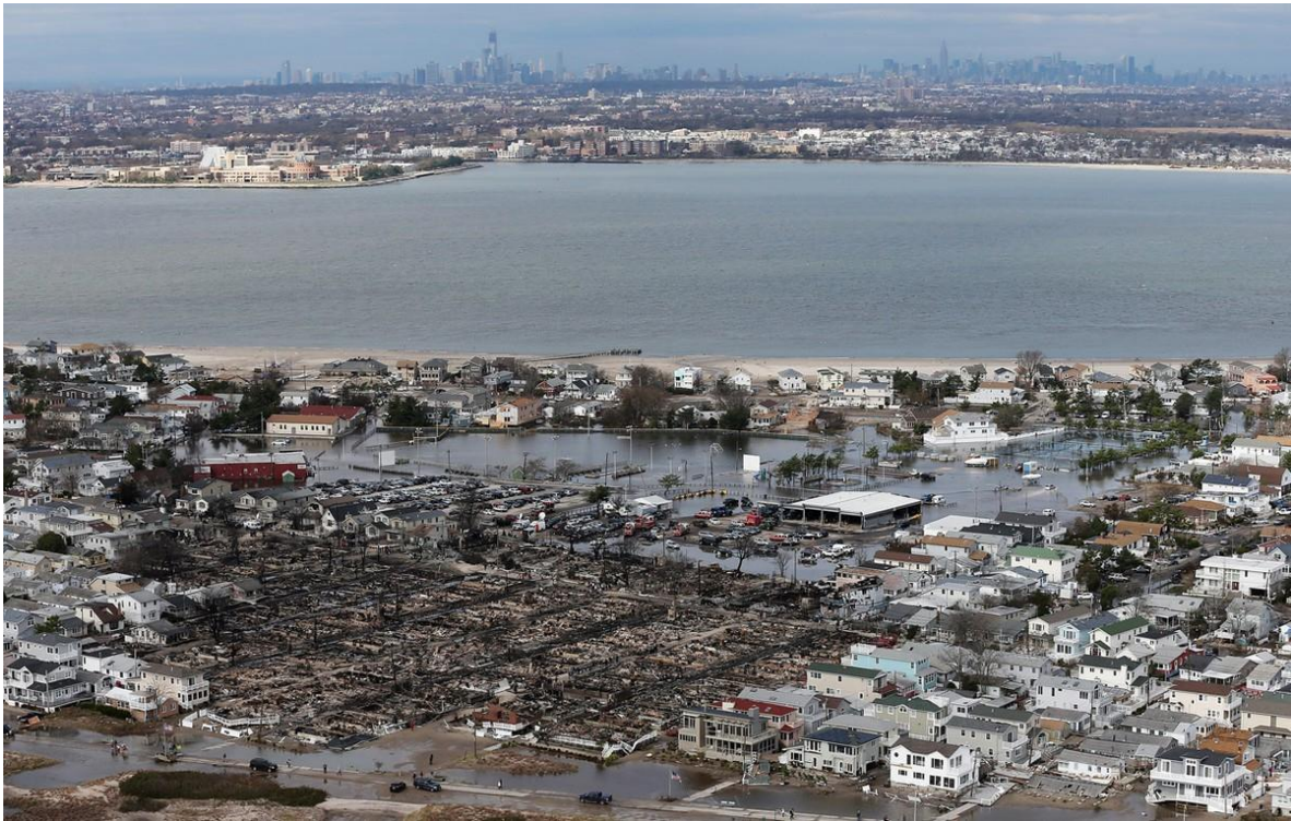
Figure 48 – The remains of burned homes in the Breezy Point neighborhood of Queens, with the Manhattan skyline in the distance after Superstorm Sandy, on October 31, 2012.
