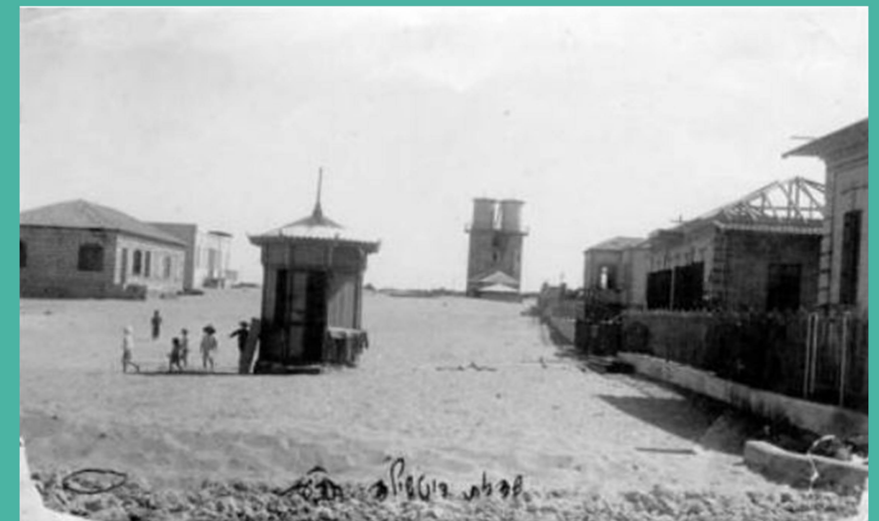
1909 The first stage of the boulevard, the lack of pavement exposes the sand flooring. A kiosk occupies the central position, and some eclectic buildings are being erected.
