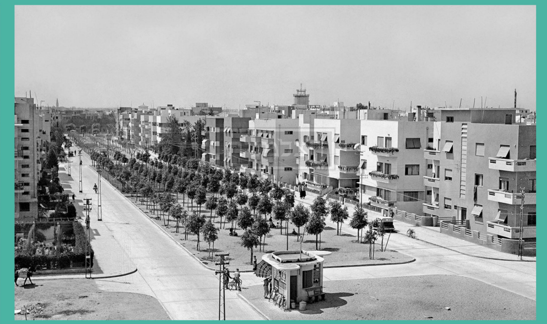
1936 A new proposal for the greenery inside the boulevard, the kiosk is introduced again. The urban grid has changed, but most importantly, the eclectic style has been replaced for Bauhaus.
