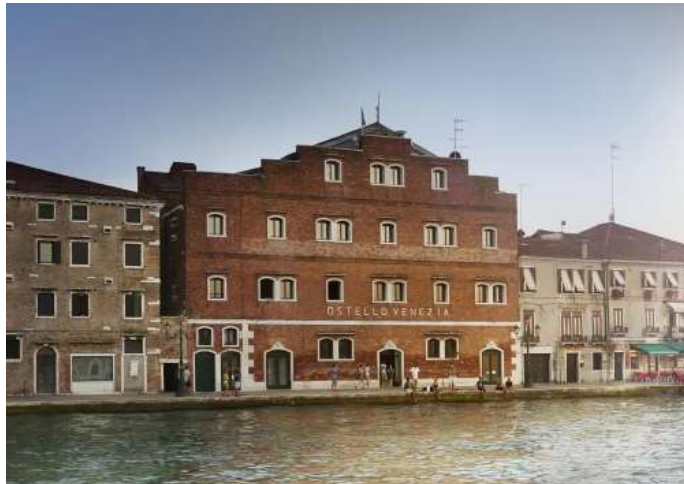
Figure III.3 Street view of Generator Venice
