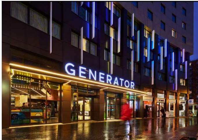
Figure III.4 Street view of Generator Paris
