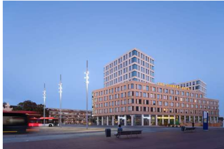
Figure III.2 Street view of The student hotel Delft
