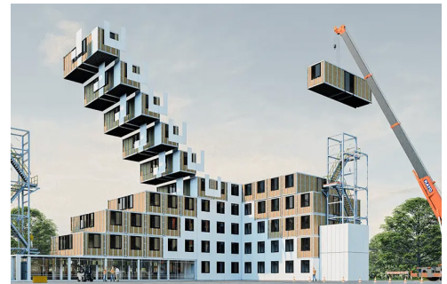
Fig. 28. Volumetric construction. Source: https://villavo.com/blog/what-is-volumetric-construction/
