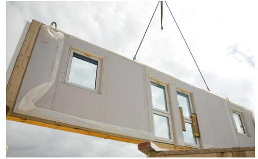
Fig. 27. Panelized construction. Source: https://www.atamate.com/atamate-blog/modern-offsite-construction-techniques-an-overview
