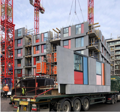
Fig. 43. Site project. Source: https://www.pbctoday.co.uk/news/mmc-news/design-for-manufacture-and-assembly/74186/
