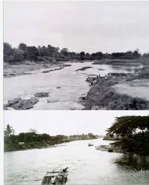
Mookervart Canal was built to connect two natural rivers and prevent flooding 1678 - 1689
