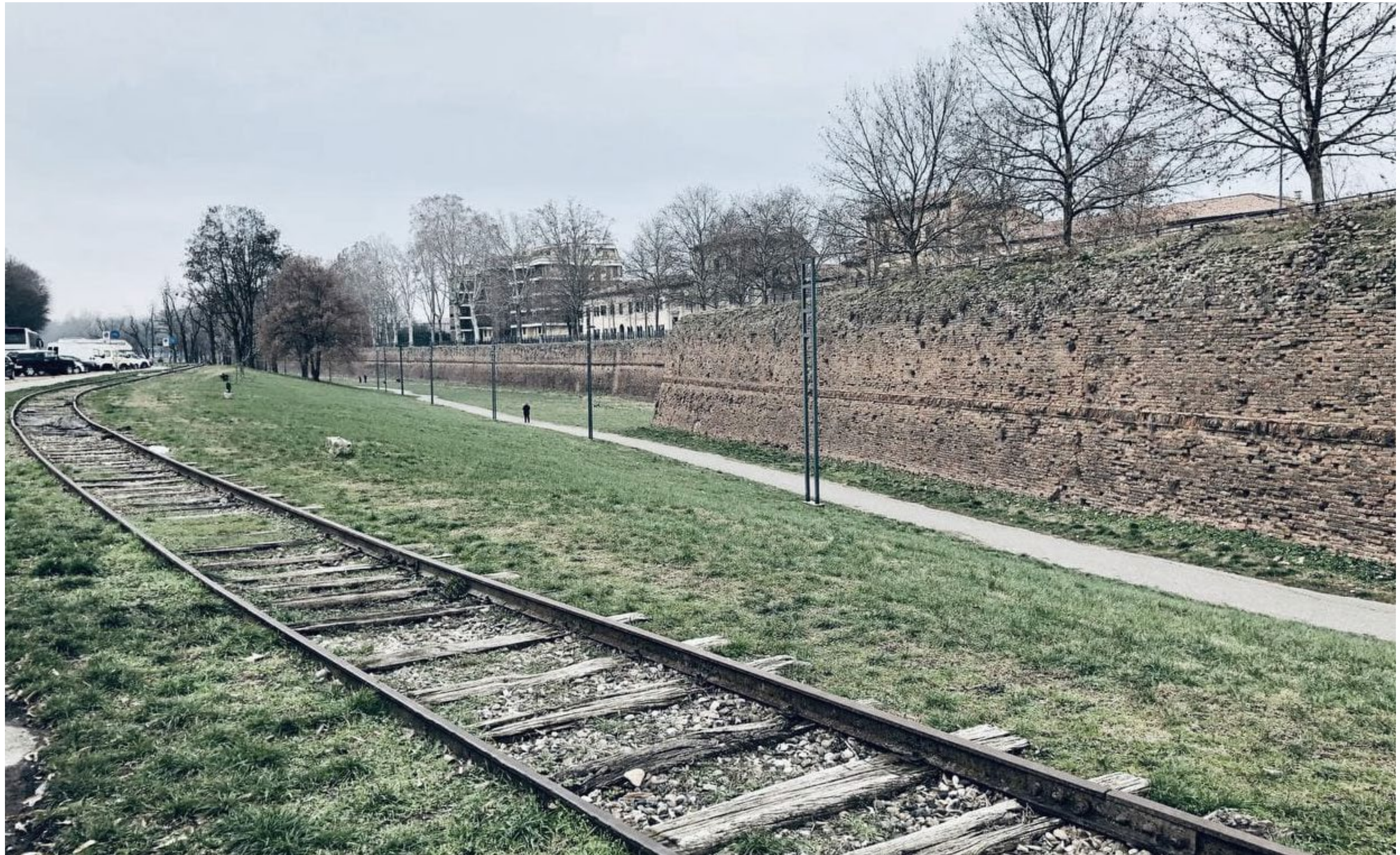
The part of old wall in Giardino Delle Mura Farnesiane
