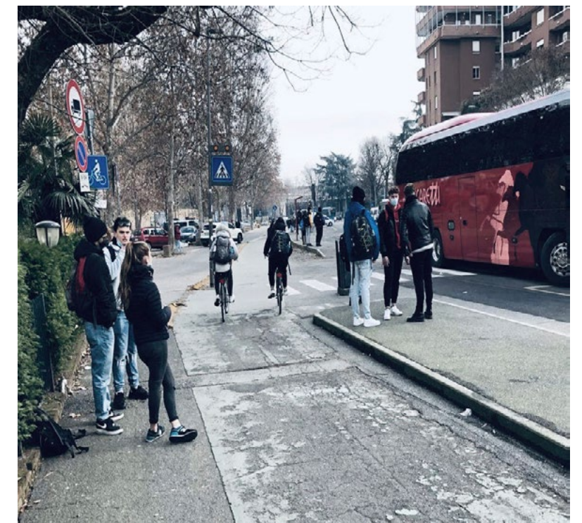
Lack of separation between users, damaged pavement
