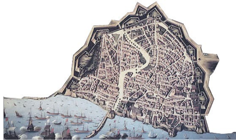
The structure of the Wall
