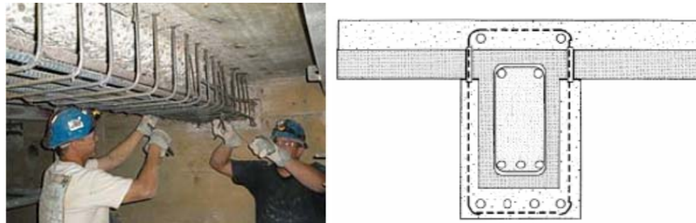
Figure 4.19 addition of steel reinforcement and concrete overlay [17]
