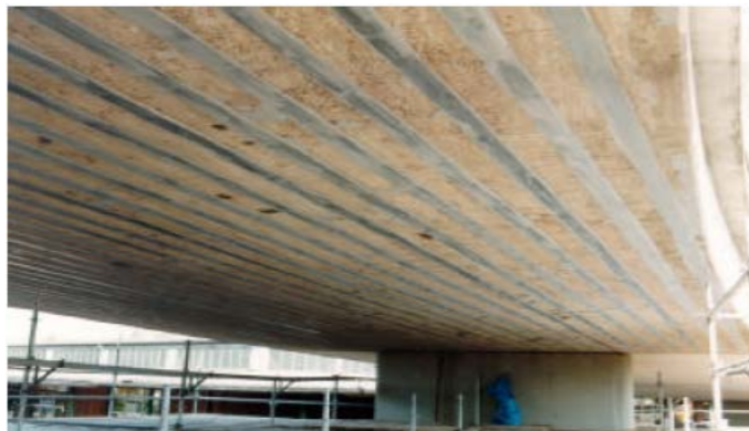
Figure 4.16 externally bonded plates using FRP [21]
