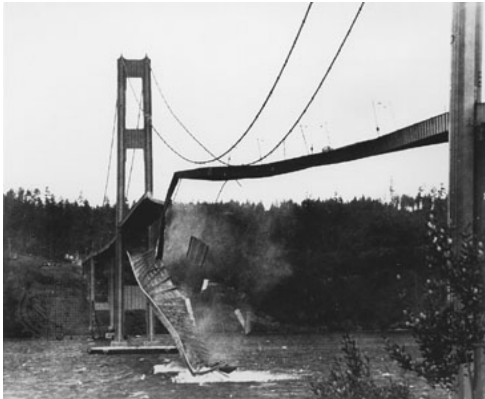
Figure IV: Takoma bridge collapse due to one d.o.f. instability
