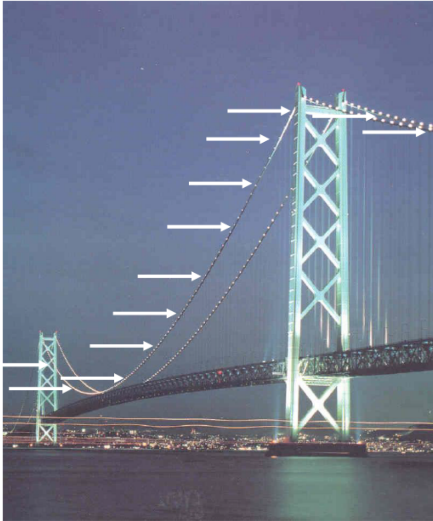
Figure III: Load transfer on Akashi Bridge
