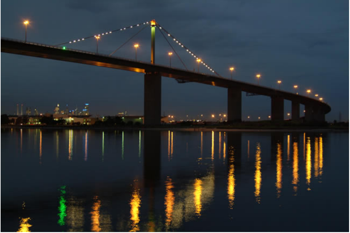
Figure 2.1: West Gate bridge
