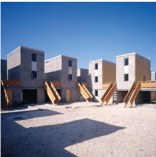
Fig. 5.3.j Quinta Monroy at the end of construction works.
