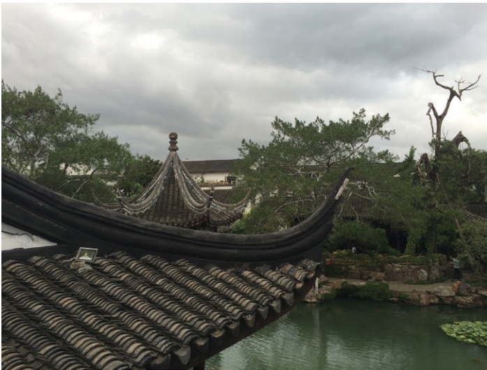
■ Fig. 2.5.ac A flared corner in the roof of the Wash Tassels Waterside Pavilion.
