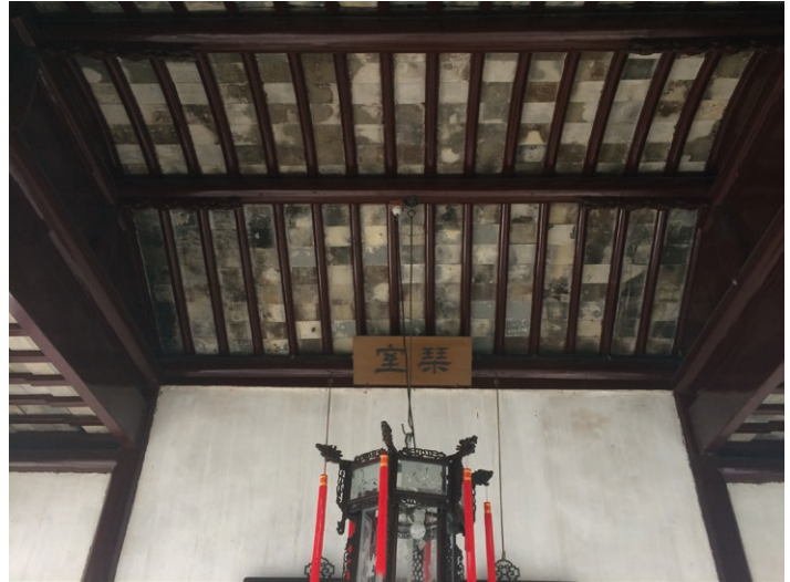
■ Fig. 2.5.ab The structure of the roof of the Zither Chamber.
