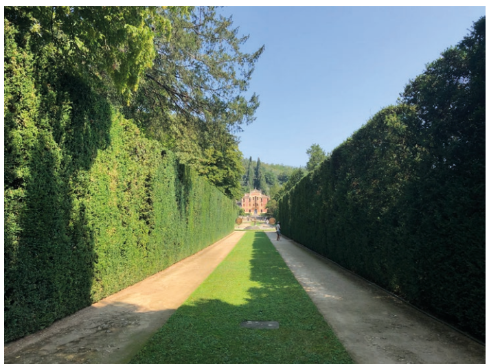
■ Fig. 4.5.l The axis of the cardo is extended indefinitely by the rows of cypresses on Mount Gallo.
