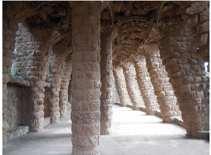
■ Fig. 5.4.d Parc Güell: the Carob's Viaduct, a cave-like structure.
