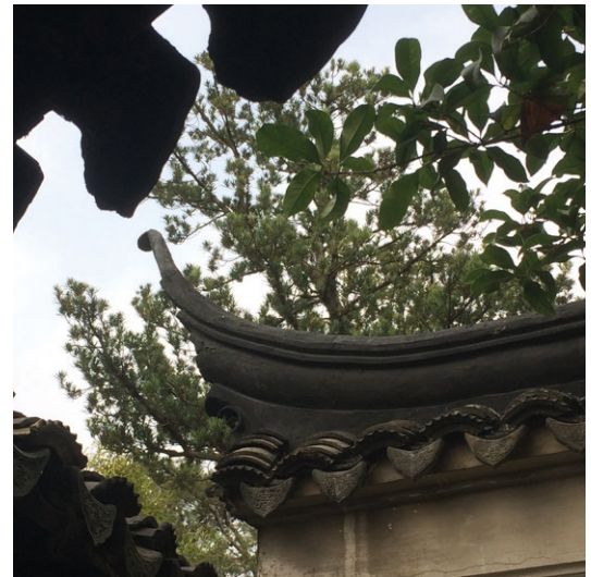
■ Fig. 2.5.ad Detail of the finials positioned at the end of the rows of tiles.
