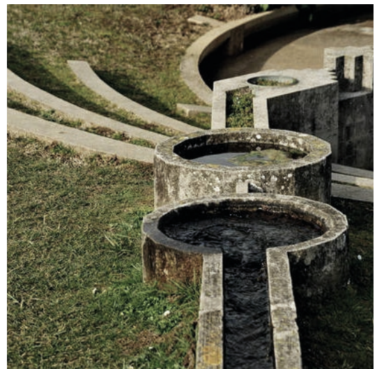
■ Fig. 5.4.ad Brion Cemetery: detail of a small fountain and concrete structures.
