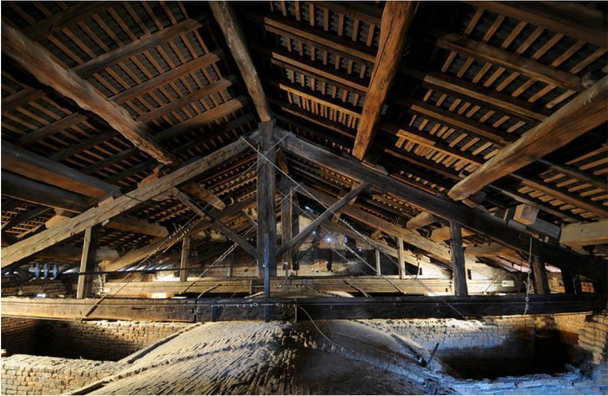
Figure 11: Trusses at the Roof of the structure
