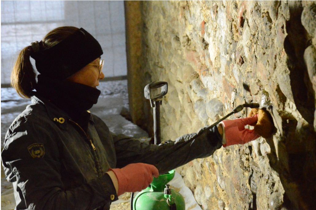
Figure 1.5: JOS method in action in Verona Arena
