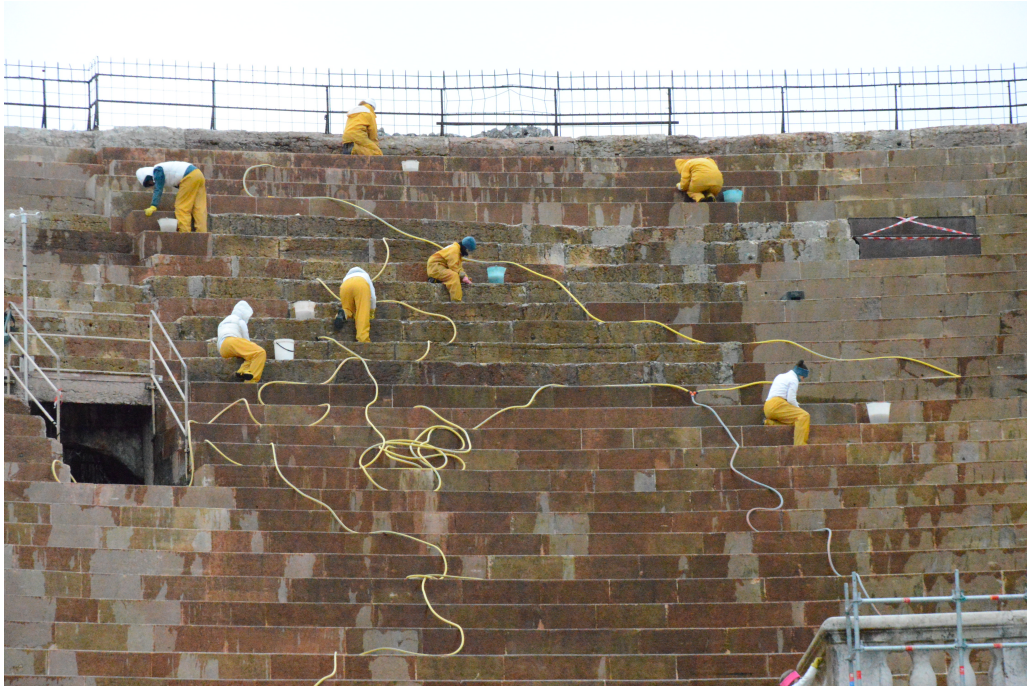
Figure 1.6: Soiling removal from the seats of Verona Arena
