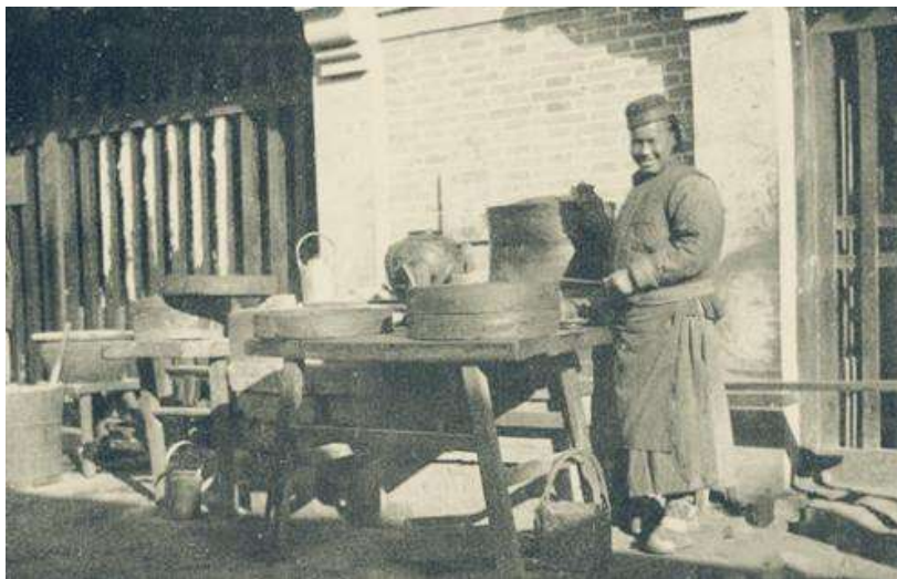
Figure 4-7 Photos of street vendors in the Qing Dynasty manifest the streets defined by walls and the position of vendors in the streets. (The shooting year unknown)
