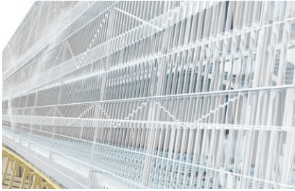
Figure 59. New Skin, Made From Corrugated Transparent Polycarbonate Panel.
