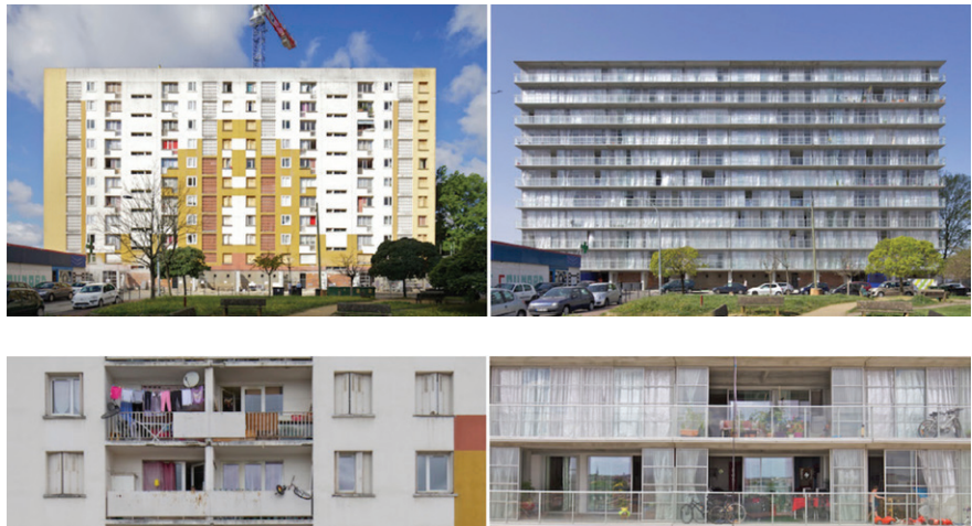
Figure 21. (a) Exterior view, (b) window before renovation, (c) window after renovation
