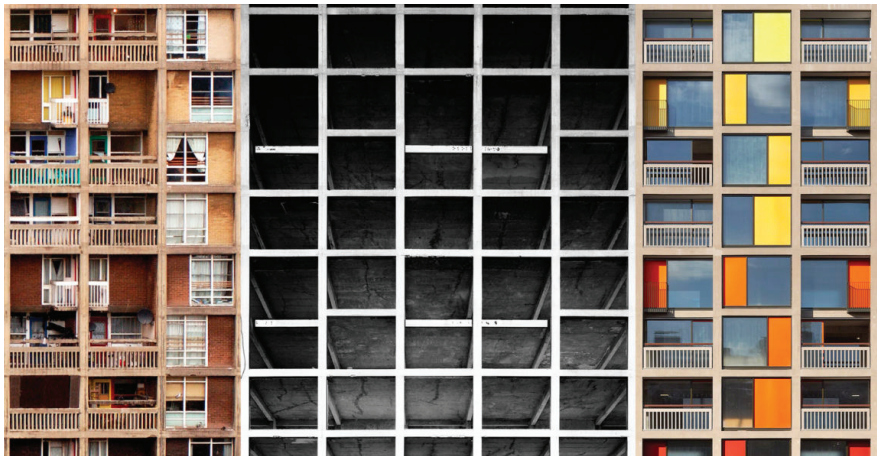
Figure 29. Facade Changing Process From Left To Right; Before, Construction, After.
