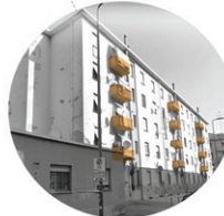
Existing Urban Facade
