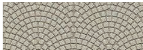
Permeable pavers used on path
