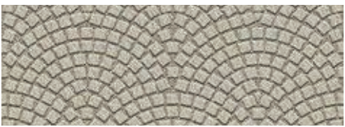
Permeable paver used in plaza
