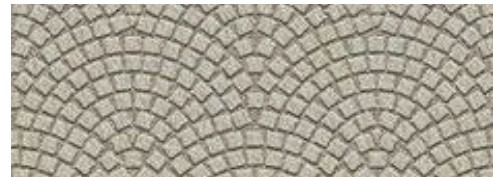
Permeable pavers used on path
