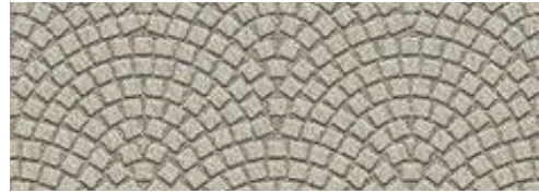
Permeable pavers used on path
