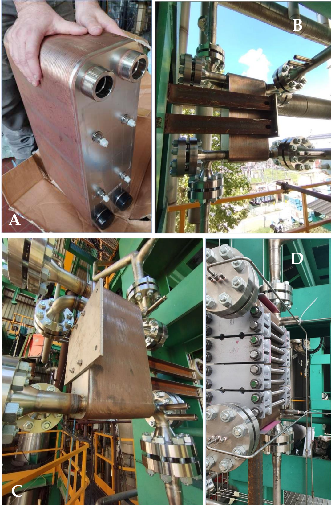
Figure 20: TEMPCO TCBC2120 “out of the box” (A), installed with metallic shield (B;C) and with mechanical guard (D)
