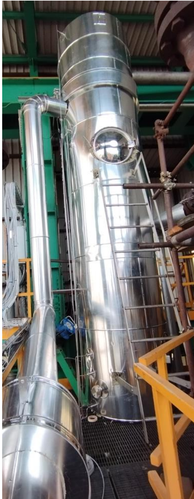
Figure 11: HX - Pool container
