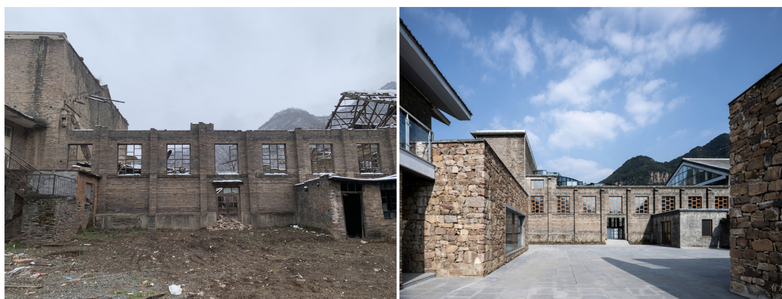
III. 39 - Before and after theater renovation
