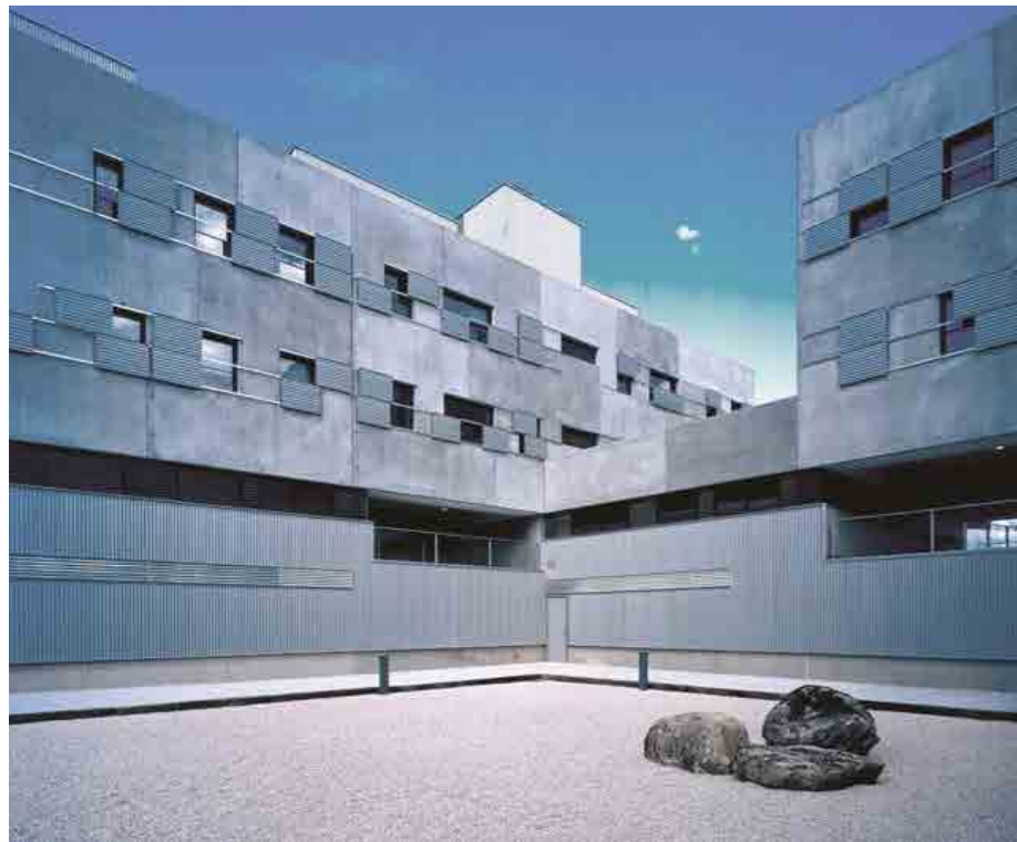
15. Photo: External view. 16. Photo: Inner view of the corner.
