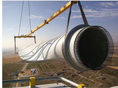
Figure 40. Turbine blades composed by glass reinforced polymer composite.
