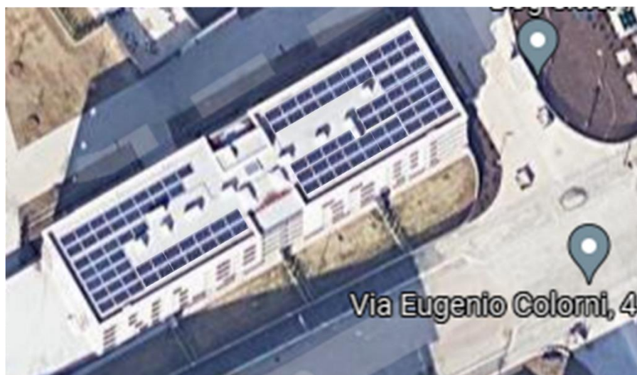
Figure 4-3– Condominium 2, UDC 1, Merezzate district, PV plant of 30 kW
