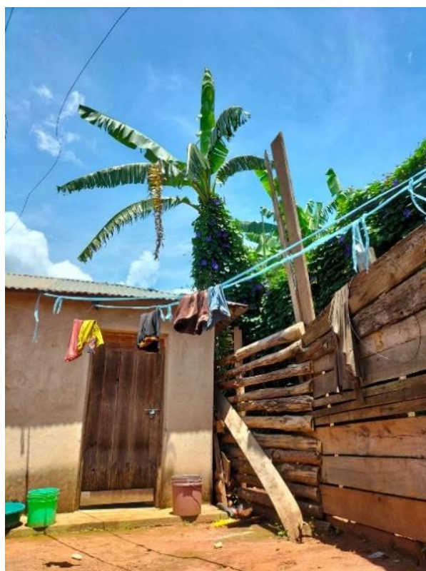
Figure 2.4: House with plaster on wall and floor.
