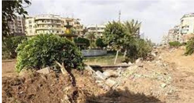
Figure 19 Example of Dredging Greenery in order to Build Roads
