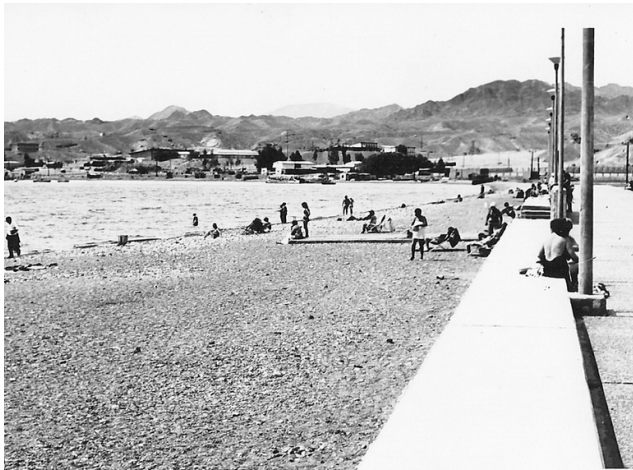
Figure 302. North coast with the new promenade, 1970. Source: Eilat's archive
