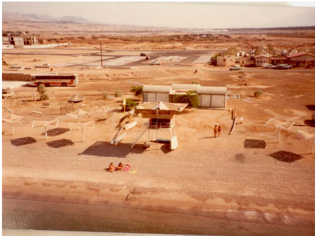
Figure 311. Aerial view at the north coast with the airport behind, 1982. Source: Eilat's archive
