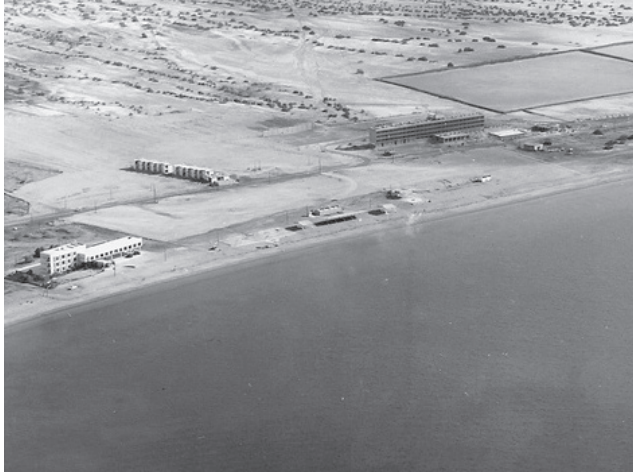
Figure 289. Aerial View of the north coast, 1965. Source: Eilat's archive
