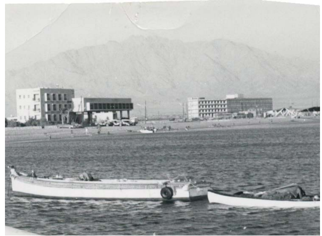
Figure 264. Eilat Hotel and queen of Sheba Hotel, 1974. Source: Eilat's archive
