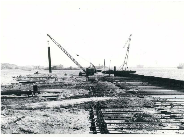
Figure x Eilat Sea Port construction, 1964. Source: Eilat's archive
