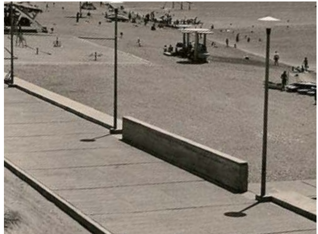
Figure 306. North coast with the new promenade, 1971. Source: Eilat's archive
