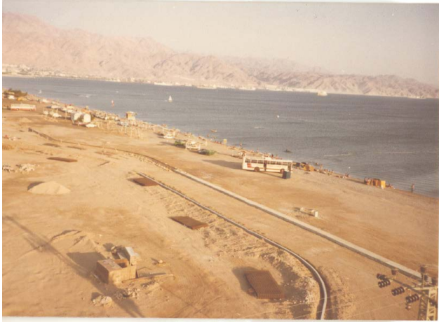
Figure 310. Construction of the promenade at the north coast, 1981. Source: Eilat's archive
