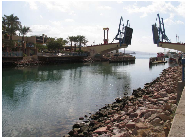
Figure x North coast bridge of the marina, 2008. Source: Eilat's archive
