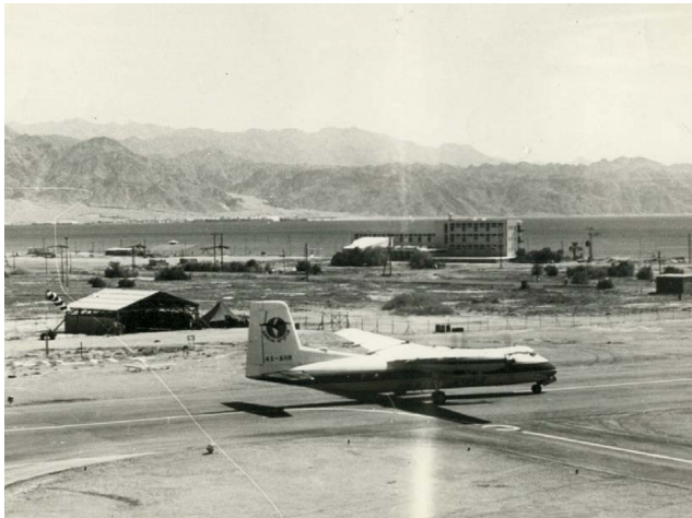
Figure 230. Plain at the airport , 1957. Source: Eilat's archive
