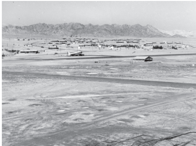
Figure 228. Eilat Airport, 1955. Source: Eilat's archive
