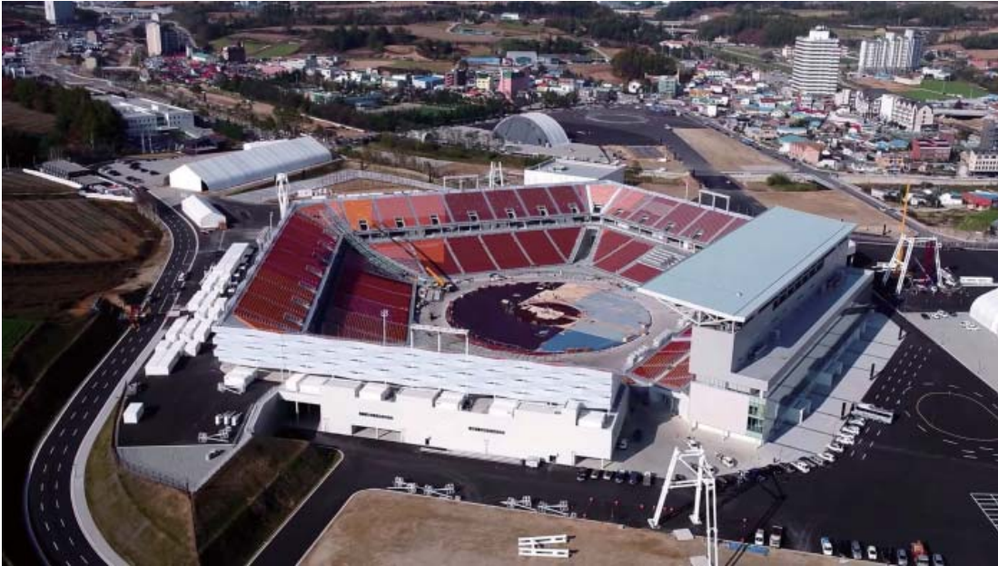
Figure 24: The temporary PyeongChang Olympic Stadium under construction.. (Source: https://www.archpaper.com/2018/02/south-korea-disposable-olympics-stadium-no-roof-heat/ )
