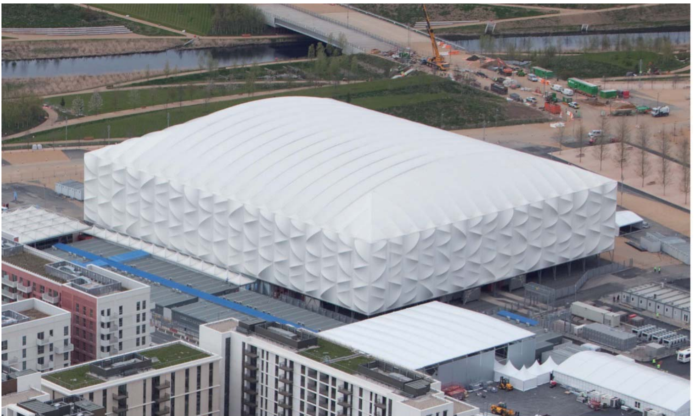
Figure 47: The basketball center at the 2012 London (Source: https://en.wikipedia.org/wiki/Basketball_Arena_(London) )
