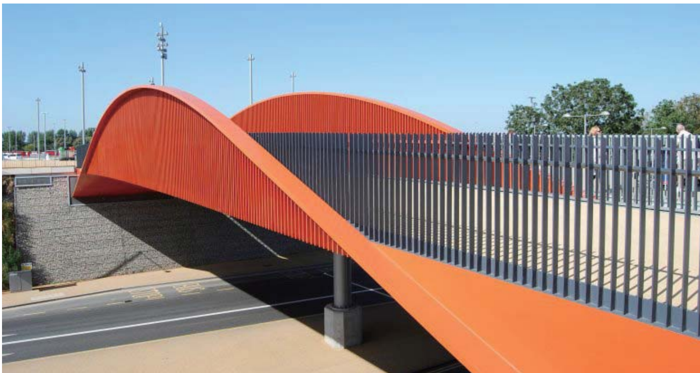
Figure 4: The temporary Olympic bridge in London 2012. (Source: https://www.lusas.com/case/bridge/olympic_park_bridges.html )
