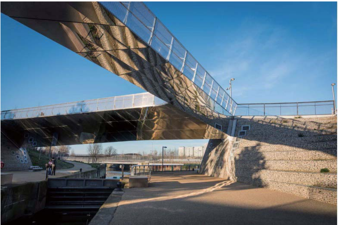
Figure 56: The temporary structures at the 2012 London Olympics (Source: https://www.akt-uk.com/projects/central-park-footbridge/ )
