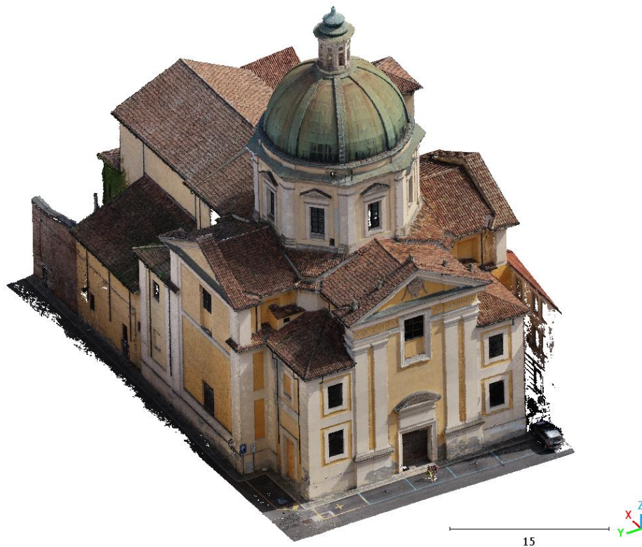
Figure 53. Integrated outdoor scene point cloud of the case study, resulting from the co-registration of UAV-photogrammetry and TLS (Gaspari et al., 2025c).
