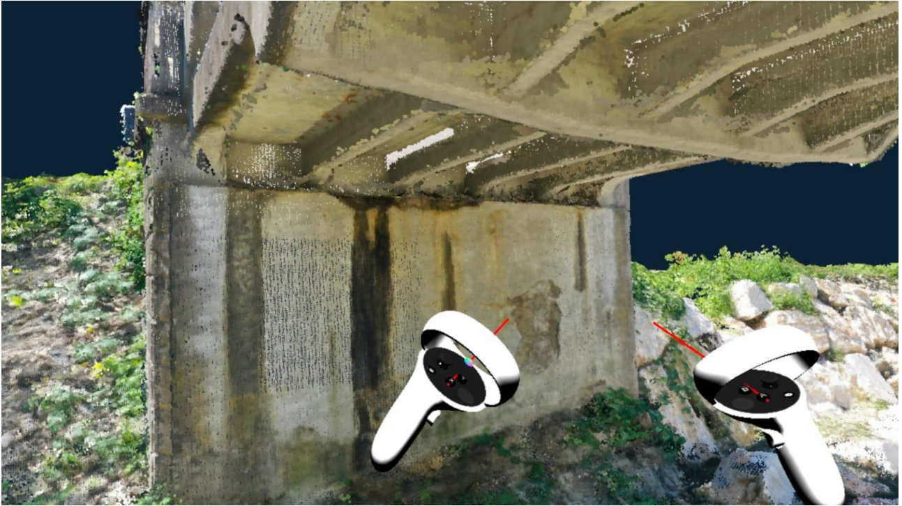
Figure 58. Screenshot of the outdoor scene point cloud of a bridge located in the Piacenza province, rendered in VR with Oculus Meta Quest 2.
