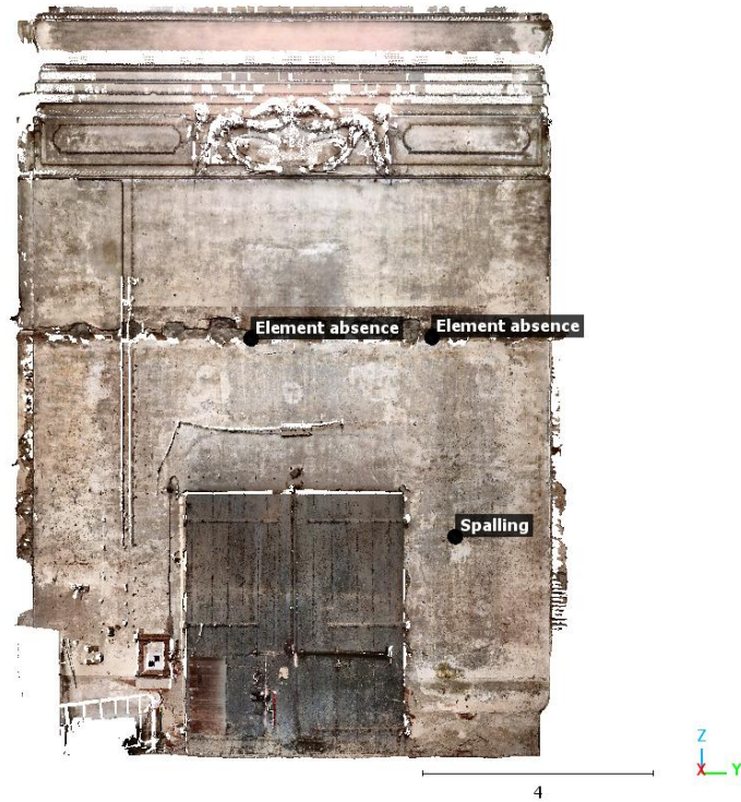
Figure 55. Exported point cloud of structural sub-element and associated annotations in the CloudCompare environment. Additional processing, meshing and rasterization can be performed to produce other products as required without having to deal with the entire point cloud (Gaspari et al., 2025c).
