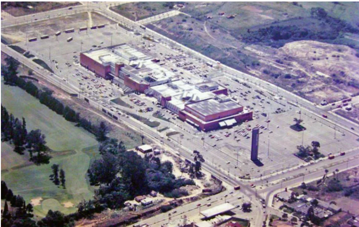
Figure A22. Construction works of Shopping Iguatemi, Porto Alegre, c. 1982 . Photographed shortly before its inauguration on 14 April 1983, the image documents the late construction phase of one of the city's first large-scale shopping centers, symbolizing the consolidation of a motorized, consumption-oriented, and increasingly "Americanized" urban model in Porto Alegre.
