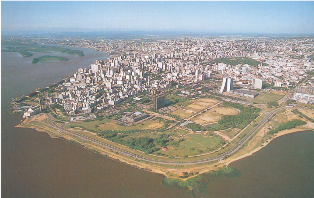
Figure 37. Aerial view of the center of Porto Alegre, showing the newly reclaimed land from the 1990s. The photograph highlights the verticalization process throughout the historic center, with the docks visible in the left background and Redenção Park in the right background. Between Redenção Park and the newly created Parque Harmonia (the green landfill area in the foreground) stands the Centro Administrativo do Estado (CAFF), recognizable by its two towers with sloped walls. In the foreground, the Edvaldo Pereira Paiva expressway connects the Gasômetro to the Praia de Belas area (located to the left, outside the frame).
