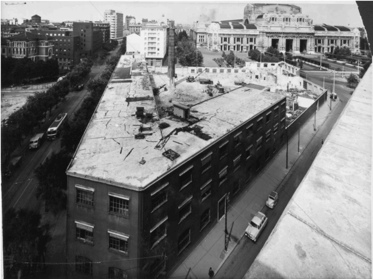
Figure A14. Demolition of the “Brusada” (June 1955), photo by Calcagni, Fondazione Pirelli. This image shows the removal of the old Pirelli factory complex (Cascina Brusada) from the intersection of Via Pirelli and Via Filzi, with excavations underway, a symbolic erasure of Pirelli’s industrial past to make way for the new corporate and architectural future.
