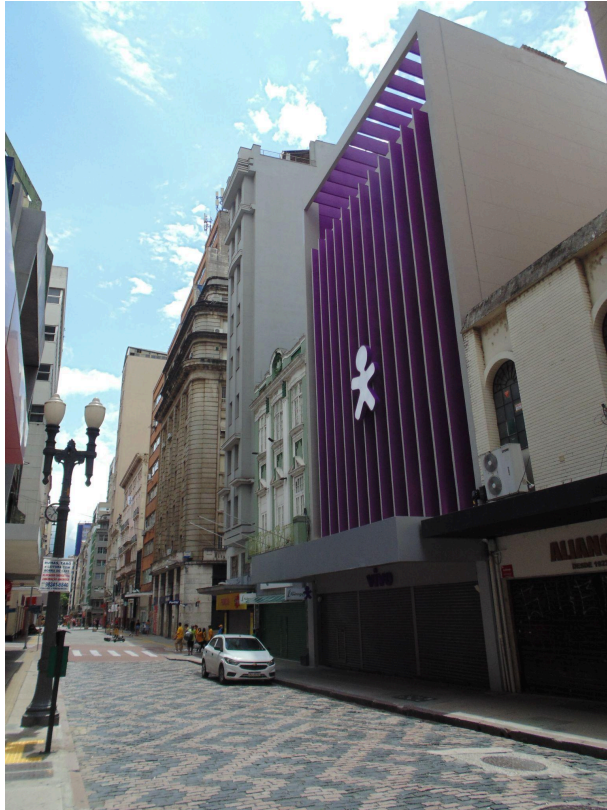
Figure A24. Rua da Praia (Rua dos Andradas), Porto Alegre. Protected historic pavement coexists with architecturally dissonant buildings, highlighting how preservation focused on individual elements fails to safeguard urban values dependent on spatial continuity and contextual relations. Source: Milena Albrecht Silveira, 2025.
