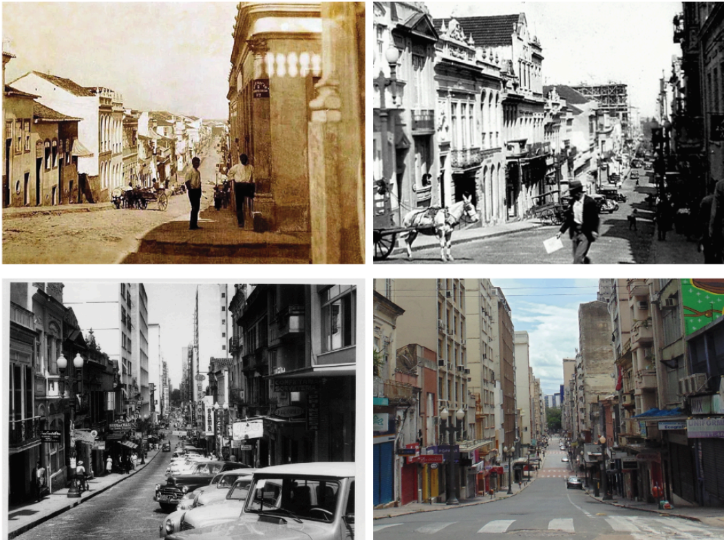
Figure 35. Rua dos Andradas/Rua da Praia in four different periods. From left to right and top to bottom, end of the 19th century, around 1910s, 1961, and 2025. Between the first and second photographs, the same houses are visible on the left side of the road. From the last three images, the lamp post is the most recognizable resemblance. The images also testify to the process of verticalization that occurred along the 20th century.
