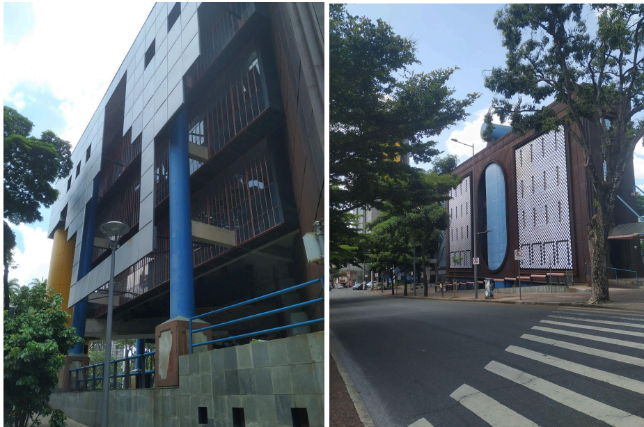
Figure A32. Prédio Rainha da Sucata (Edifício Tancredo Neves), Praça da Liberdade , Belo Horizonte, Brazil. Designed by Éolo Maia and Sylvio de Podestá in the 1980s, this post-modernist building is an example of contested meaning within the city's heritage discourse. Its eclectic mix of materials, forms, and colors, elicited sustained criticism in public and professional media, often framed as visually discordant or aesthetically deficient. The popular nickname "Rainha da Sucata" reflects how media and cultural narratives can delegitimize architectural expression, positioning certain modernist/post-modernist works as failures or regressions rather than as legitimate contributions to urban identity.
