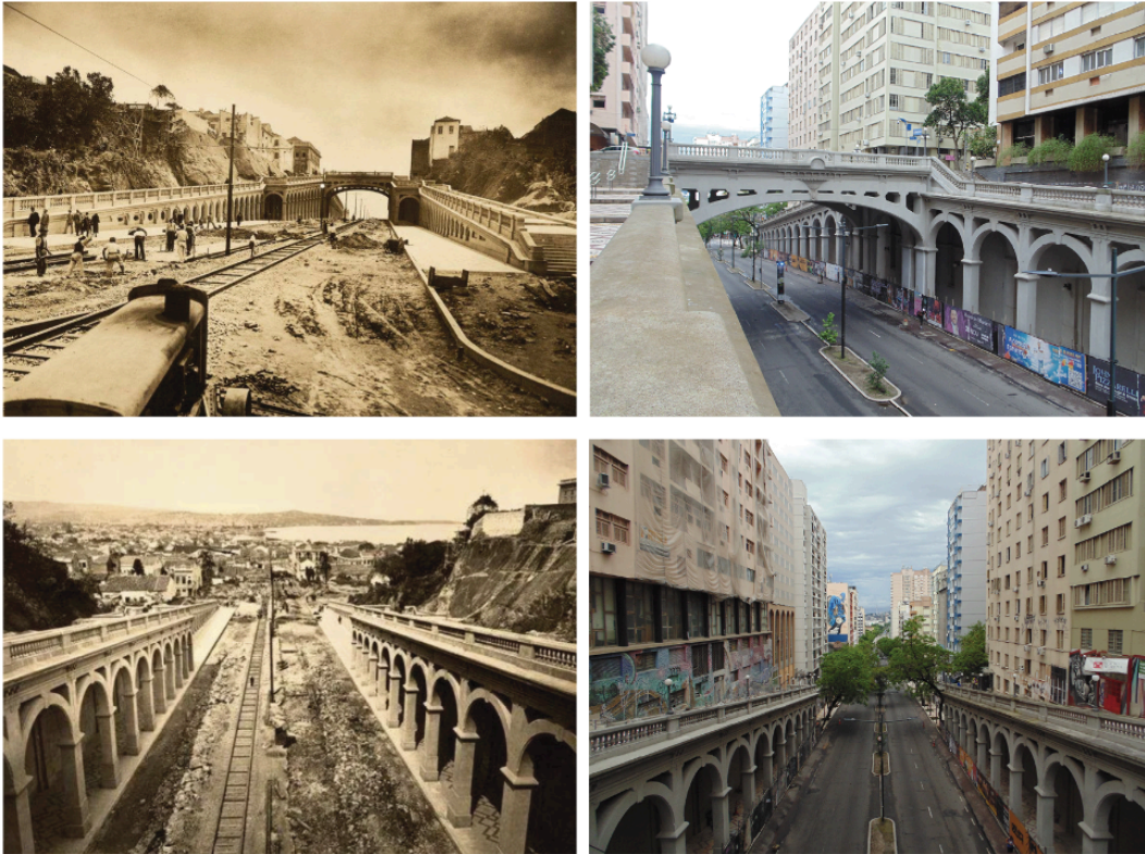
Figure 27. Opening of Borges de Medeiros Avenue and construction of the Otávio Rocha Viaduct in the late 1920s. These photographs capture a pivotal moment in the city's transformation: the erasure of older, hilly topography and the imposition of a new urban geometry, a broad boulevard carved through the "morrinho" that once separated the historic core from the southern zones. The newly laid tram tracks suggest an early commitment to modern mass transit, signalling the ambition not only to connect disparate zones but to reimagine the mobility and social rhythms of Porto Alegre. Comparison with 2025 photographs where it is possible to see the urban palimpsest as a result of the plans.
