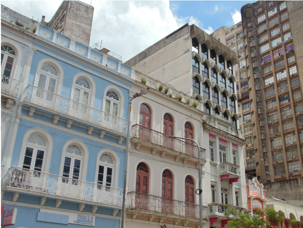
Figure 1. Porto Alegre's urban palimpsest in the historic center, where different styles coexist in the same area. Photograph taken at Rua José Montauray.
