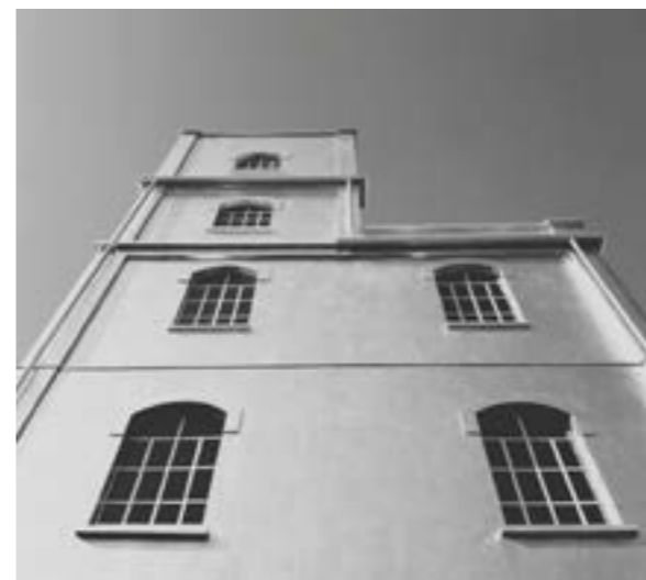
Fig.25: Present picture of Fondazione Prada as a landmark in the branding of the area
