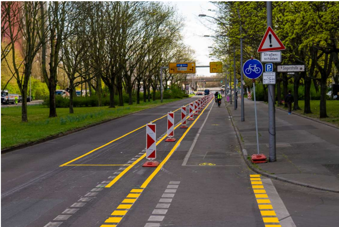
Figure 37 Berlin pop-up cycle path, with protection provided by both delineators and the row of parked cars shifted to the left
