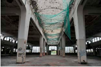
F.1.7 - Building 1 - Car storage
