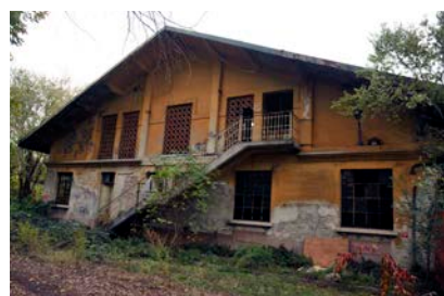
F.1.9 - Building 3 - Pre-slaughter stalls
