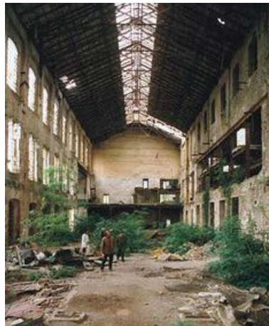
F.3.8 - Internal view, pre renovation
