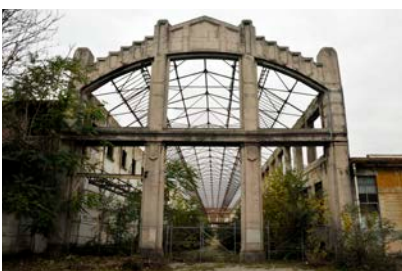
F.1.14 - Building 0 - Galleria
