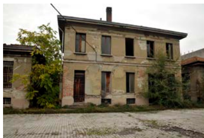
F.1.12 - Building 17 - Offices and storage
