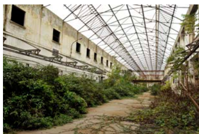
F.1.15 - Building 0 - Galleria, internal space
