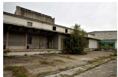
F.1.13 - Building 19 - Cold rooms
