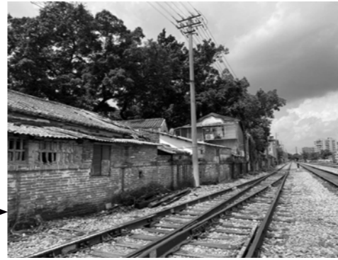
railway level is same as ground level
