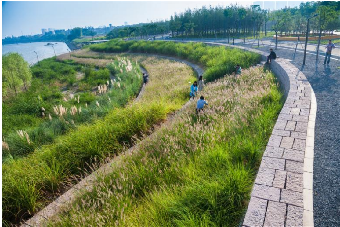
Figure 1.12. The park's terraced system. Retrieved from: https://www.turenscape.com/project/detail/4629.html .
