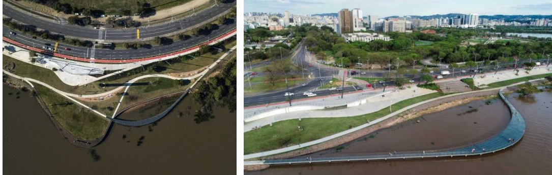
Figure 1.20. Riverside landscape platform and corridor design (Leonardo Finotti, Arthur Cordeiro) The scenic dimension of the estuary will be enhanced by the provision of a qualified stage for its appreciation. The stairways that run along the project provide the perfect seating area for the glorious sunset, “the most beautiful one in the world”.
