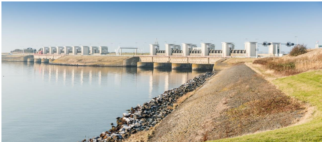
Figure 1.8. The sluices at Den Oever. Retrieved from:
