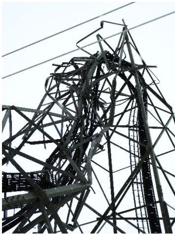
(a) Tower n22, upper area.
