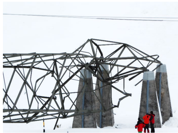
(b) Tower n25, basement.
