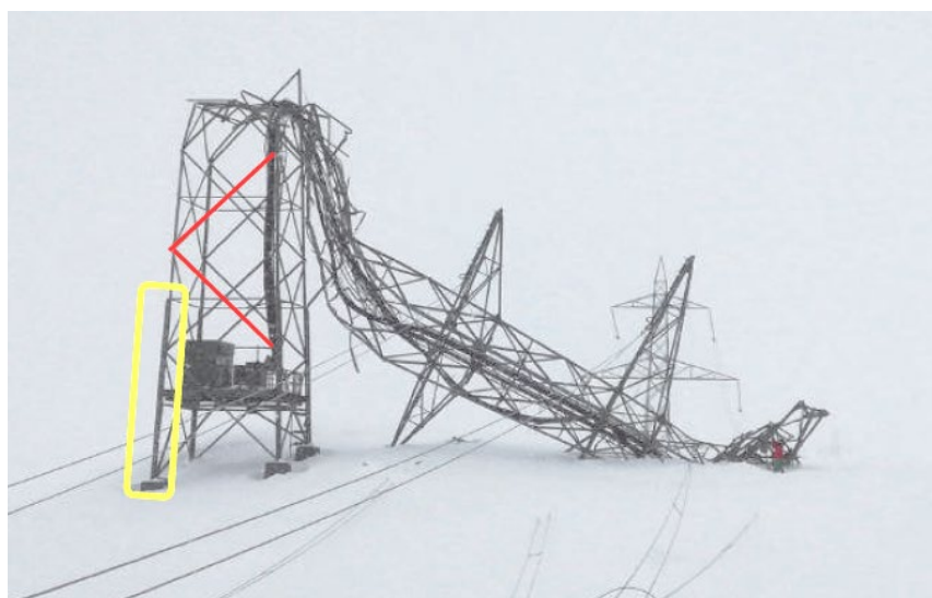
Figure 6.3: Tower n22, reinforcements made at the basement level (yellow) and at the diagonals (red) [11].
