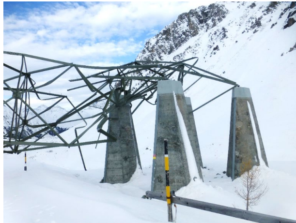
Figure 5.54: Foundations of mast n25, unaffected by the collapse (source Swissgrid ).
