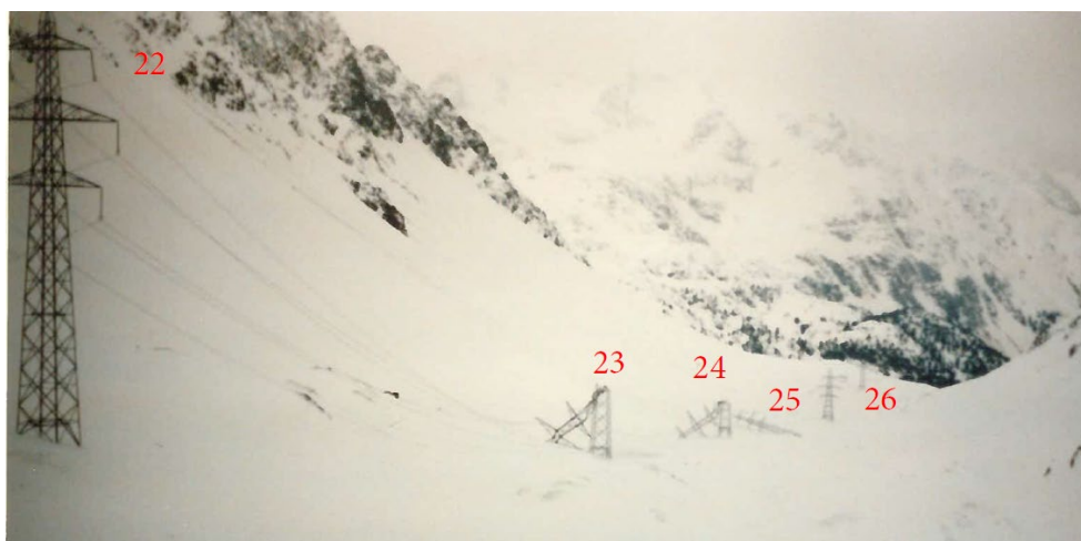
Figure 0.8: Towers n22, n23, n24 and n25 after the event in 1986 (source SwissGrid ).
