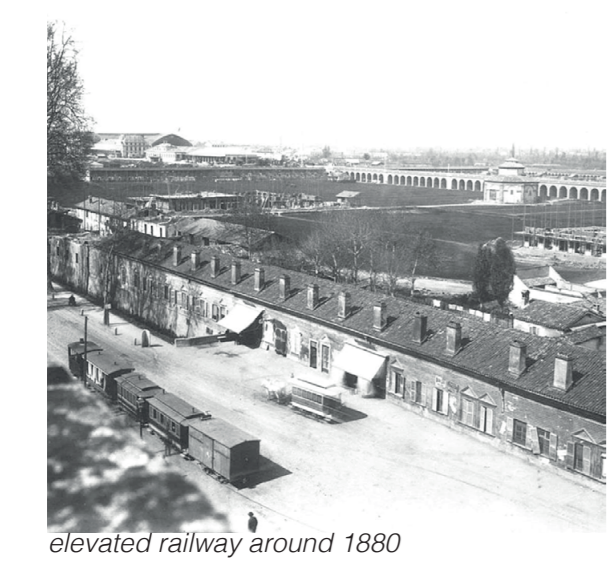
elevated railway around 1880
